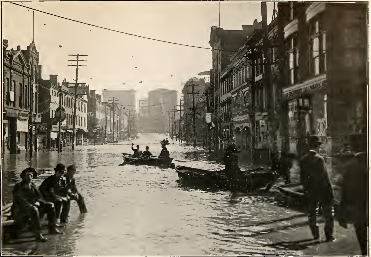
FLOOD OF MARCH 15, 1907. Federal Street, N. S., looking south from Lacoek Street.
